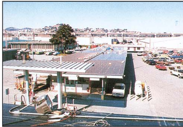
CTEM base sheet is installed over roof insulation.
